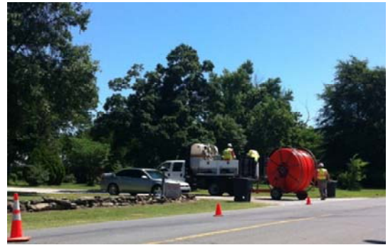
A construction crew in Warner, Okla., deploys new fiber that will bring broadband service to Connors State College.
