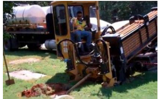
A member of Maryland DoIT drills a site in La Plata, Md., to deploy fiber as part of the One Maryland Broadband Network project.
