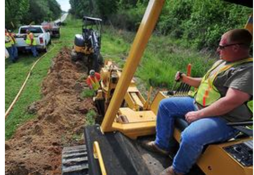
Workers for Troy Cablevision dig a trench to install a broadband cable in Ozark, Ala. The project has connected 49 community anchor institutions through June 2012.
