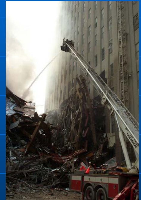
Washington Street view of Verizon's West Street building after the collapse of 7 WTC. Numerous building breaches on floors 1, 2, 4, 7, and 9 caused by the collapse.
