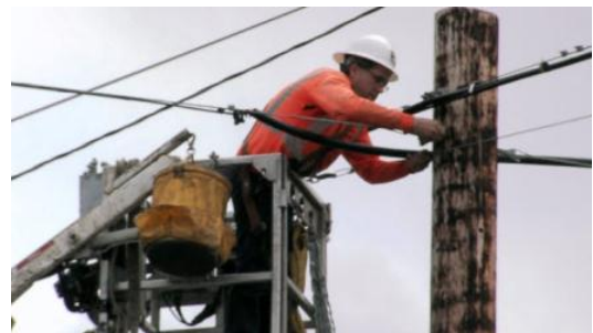
A construction worker strings fiber-optic cable for the NoaNet project.
