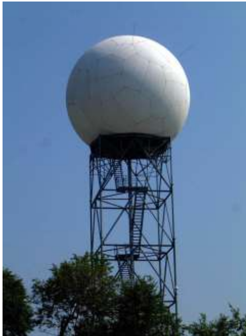
Figure 3. Typical NEXRAD Installation
