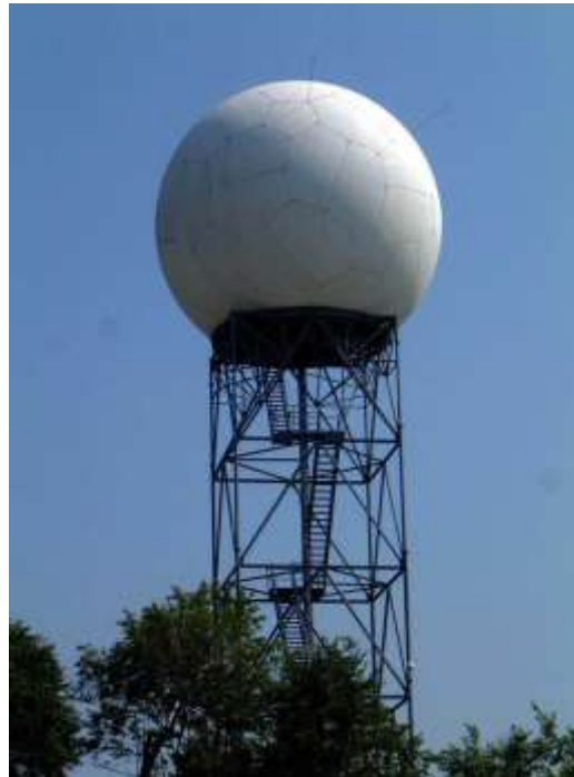
Figure 6. Typical NEXRAD Installation
