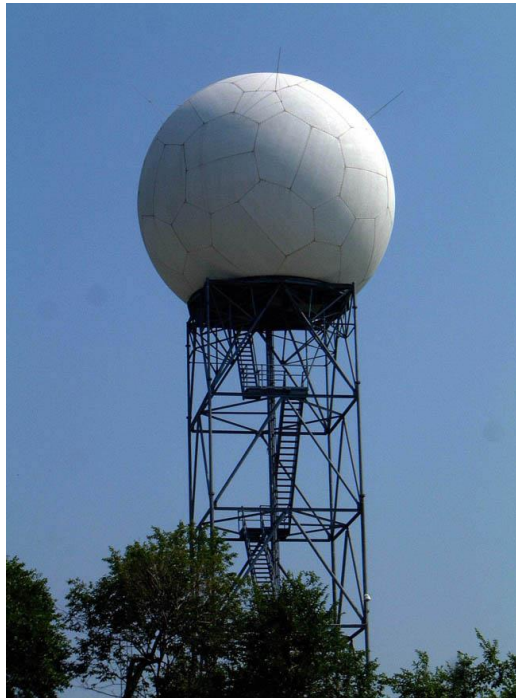
Figure 6. Typical NEXRAD Installation
