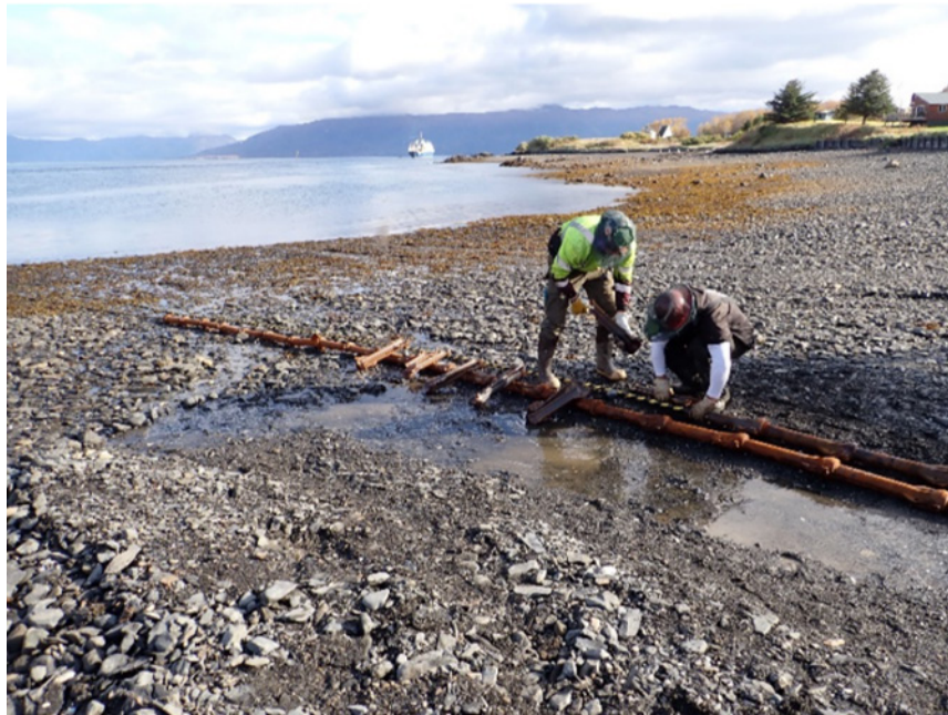
Figure 2-4. Typical Landfall Installation Showing Split Pipe Articulated Armor
