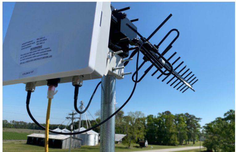
TVWS CPE installed near Engelhard, NC.
